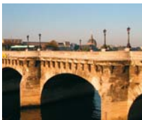
le pont luh pohn bridge
